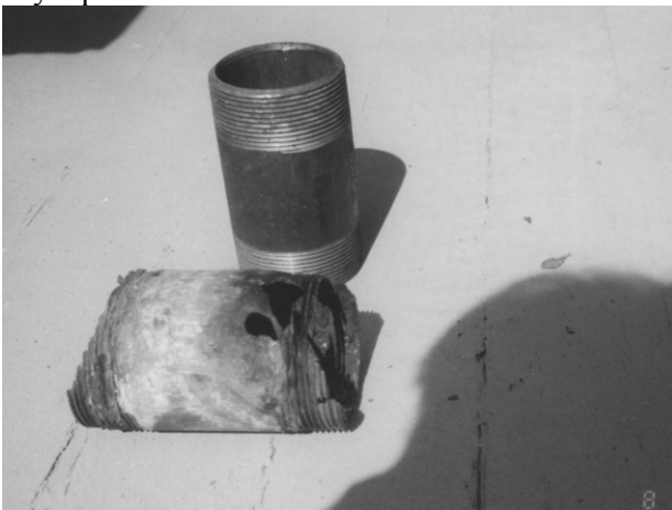
New replacement for pipe in boiler return line
