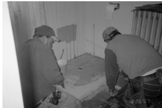
Repairing bathroom in the museum
