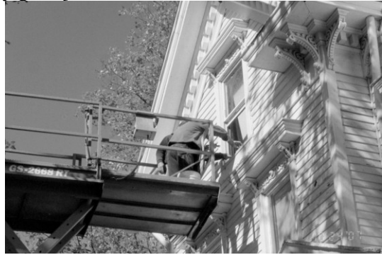
Lyle Walters & Vernon Smith repairing attic window sills
